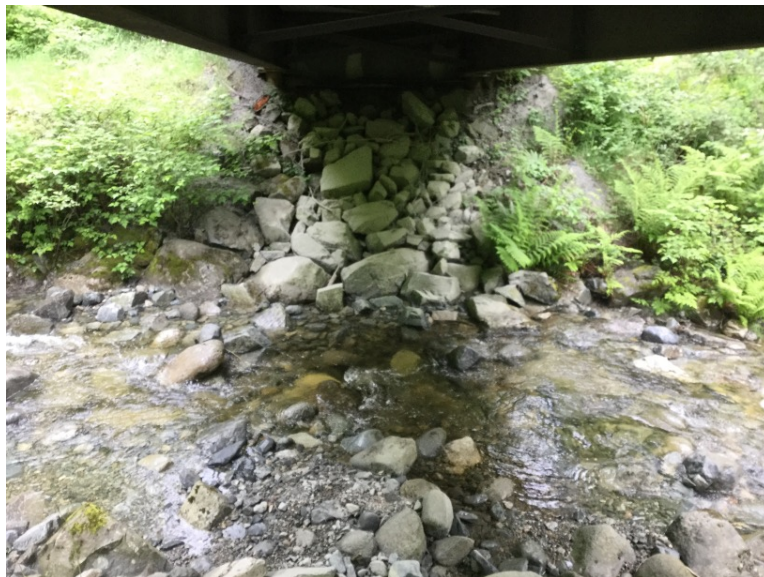
Left Bank Abutment when facing downstream
