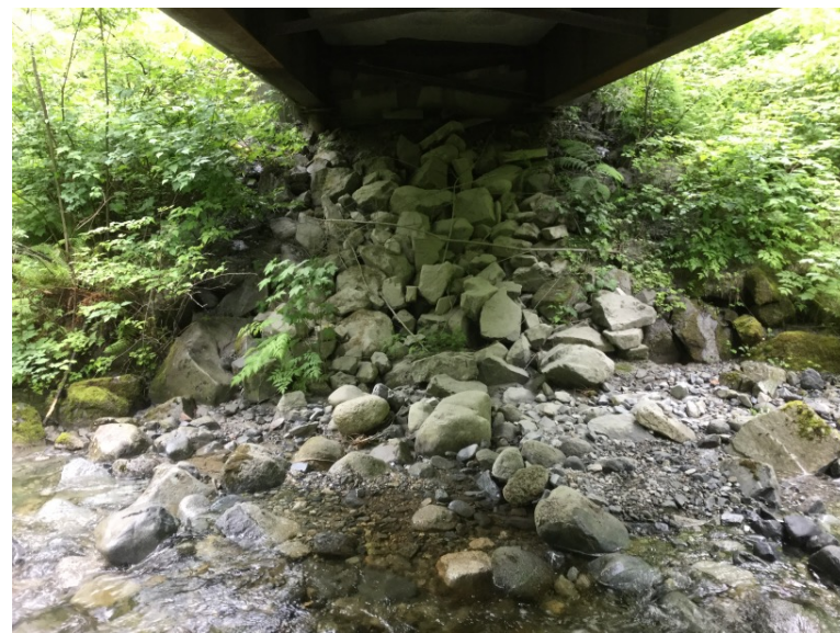
Right Bank Abutment when facing downstream
